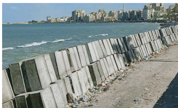
Concrete walls built in Alexandria to protect the city from the rising sea. Photo: Amira Sayed
