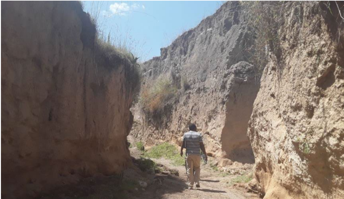
Figure 17. The gullies are unusually deep to treat conventionally
