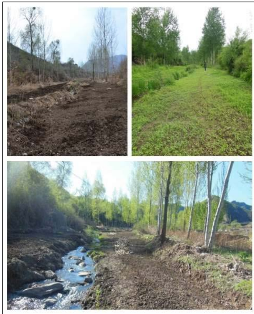
Figure 10. Buffer Strips before and after construction in Xiaowopu Village, Miyun
